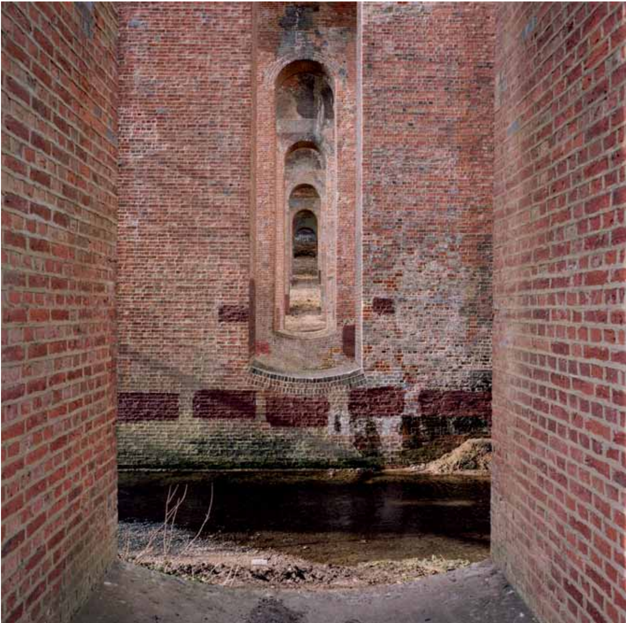
Dollis Brook Viaduct, Finchley, Barnet, London
